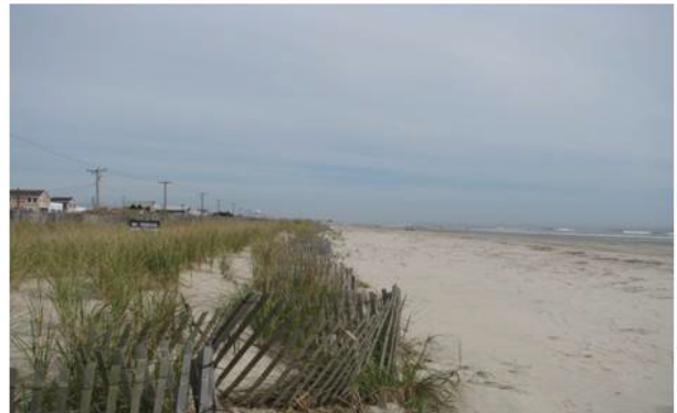
Figure 337: Historically, this site is known for its low elevation and narrow beach. The gradual decline in sand volume is evidence for a limited supply reflecting this low, narrow part of the barrier system. However, the 2009 replenishment sand has added 70 feet of shoreline as well as 32.95 yds 3 /ft of sand.
