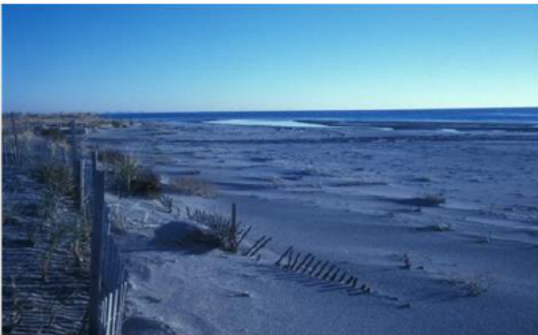
Figure 333: There have been three State/locally sponsored projects in Strathmere (1984, 2001, and 2009) that have enabled dune and beach growth for the 25 year period. Overall cumulative sand volume gains of 61.49 yds 3 /ft and a shoreline advance of 109 feet were recorded. Photo on left taken in 1988. View to the north. Photo on right taken October 10, 2011. View to the north.
